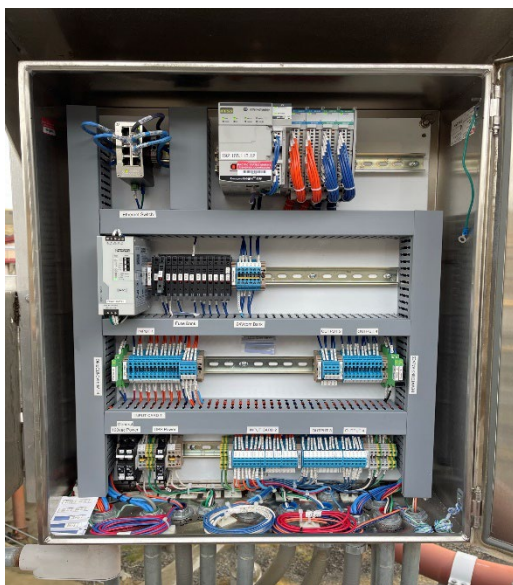
Figure 23. PLC upgraded at LMJ
