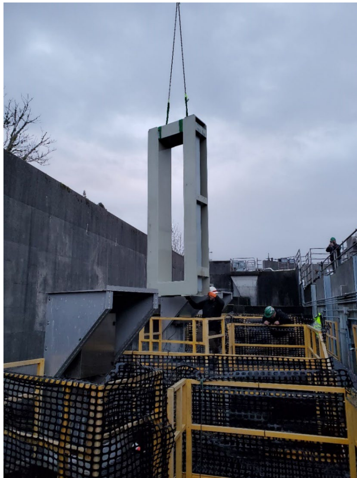
Figure 2. Installation of a slot antenna at Washington Shore serpentine weir (BO4)
