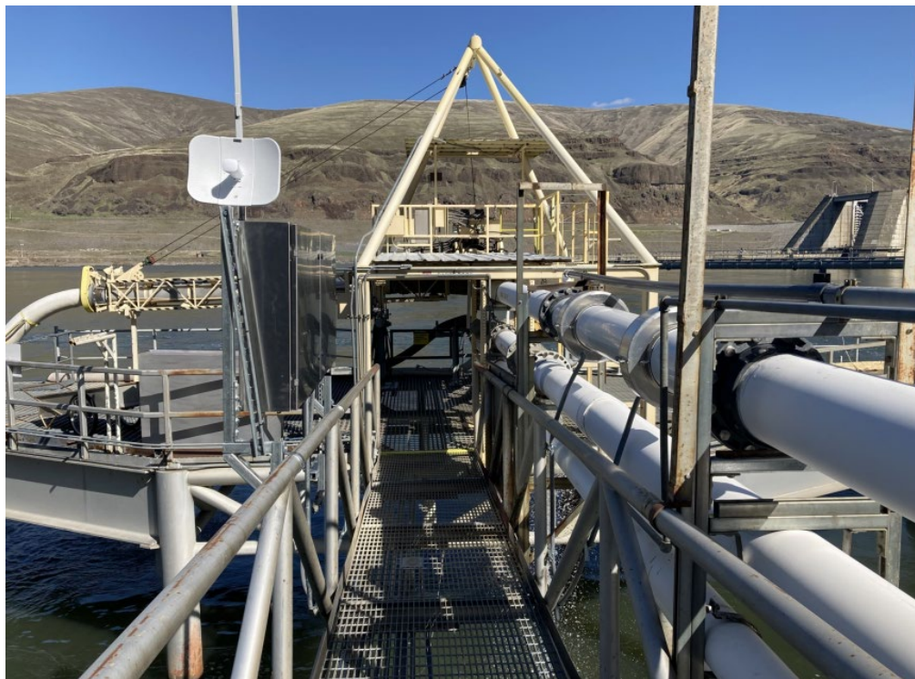
Figure 31. PIT tag antenna infrastructure including wireless Ethernet antenna dish (upper left) at GRJ barge dock
